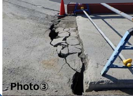
② : Unit 5 south side ramp Road subsidence/ground subsidence, etc.
