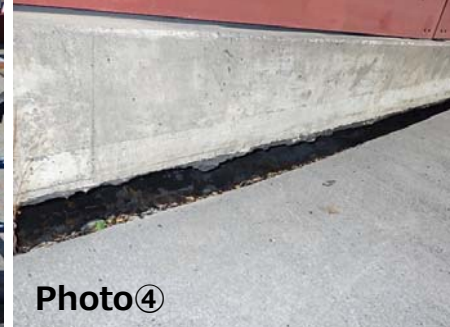
② : Unit 5 south side ramp Road subsidence/ground subsidence, etc.
