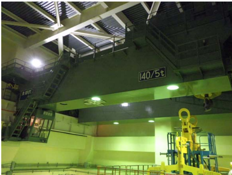
Ceiling crane in the cask loading/unloading area
