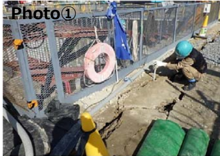
① Unit 5/6 seawall yard
