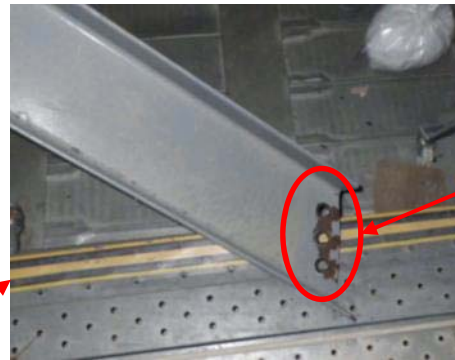
Bolts at the joint ruptured
