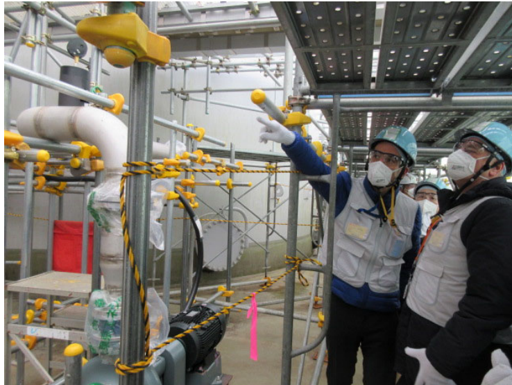
K4 tank area
