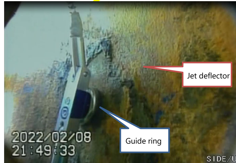
Installed 3 rd guide ring (Installed at 9:49 PM on February 8)
