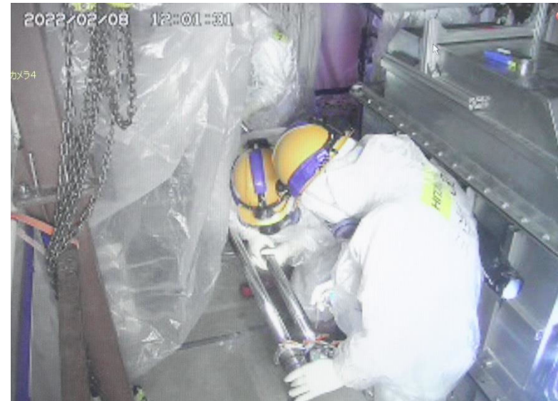
Work in the area in front the X-2 penetration (2) 10
