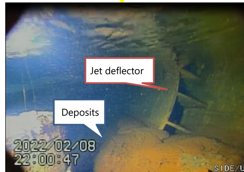
Deposits near the 4 th jet deflector
