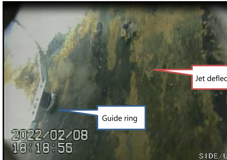
Installed 1 st guide ring (installed at 6:18 PM on February 8)
