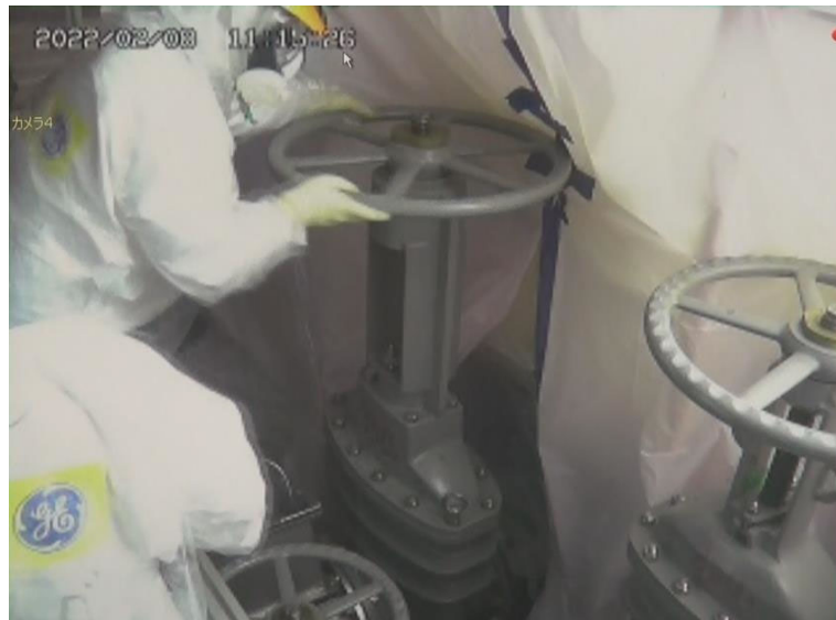
Work in the area in front the X-2 penetration (1)
