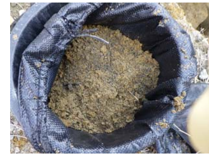
Excavated soil (around G.L.-2.6m) 11/10 : Excavation of surface layer commences 11/11 : Excavated to G.L.-1m~2m 11/12 : Excavated to G.L.-2.8m
