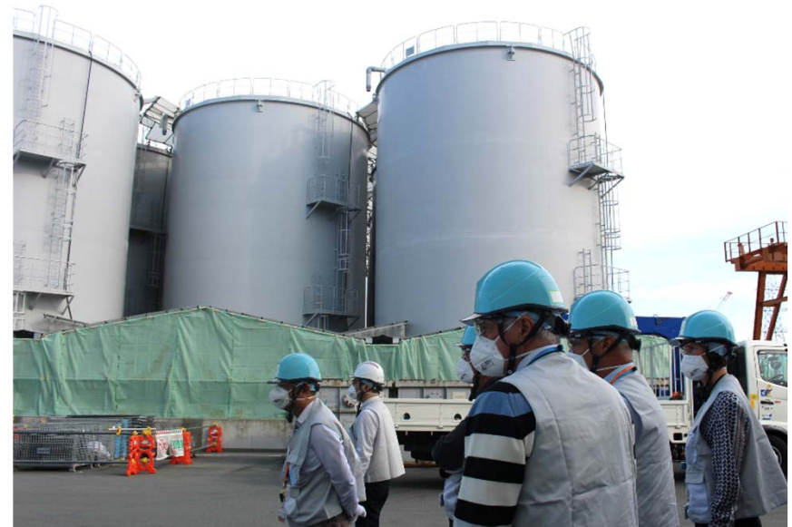
K4 tank area
