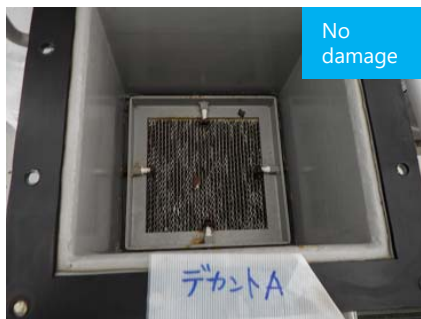
Existing ALPS decanting tank A
