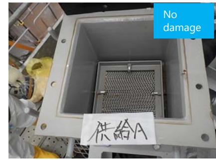
Existing ALPS feed tank A
