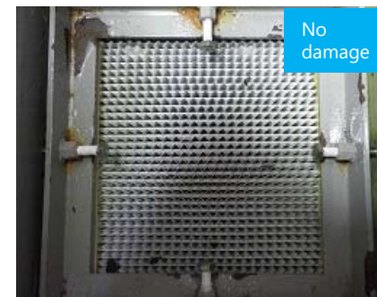
Existing ALPS water discharge tank (reposted)
