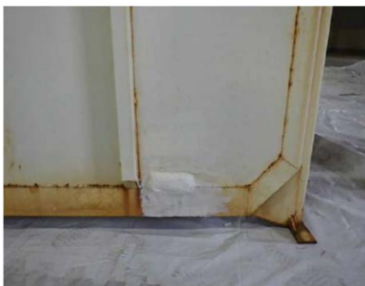
Figure 1. Corrosion repair
