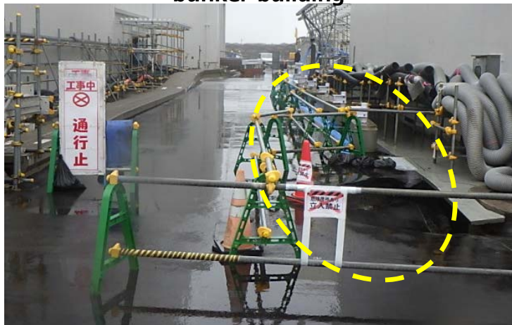
② Road on the north side of the site bunker building
