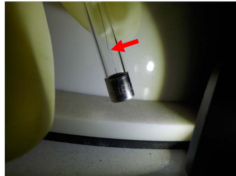
②Aforementioned blown fuse (arrow indicates severed element)
