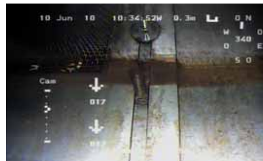
Movable weir bolts (bottom right of northwest side)
