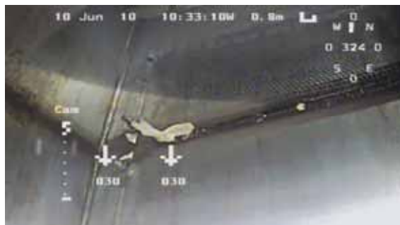
Front of skimmer surge tank entrance (northwest side)
