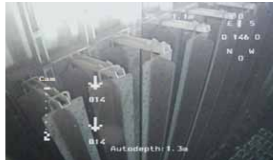
Control rod hangers (northeast side)
