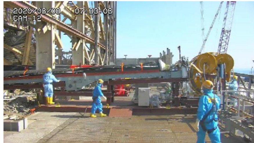
3. Inspection of insertion equipment before cover bag insertion (Photo taken on June 8)
