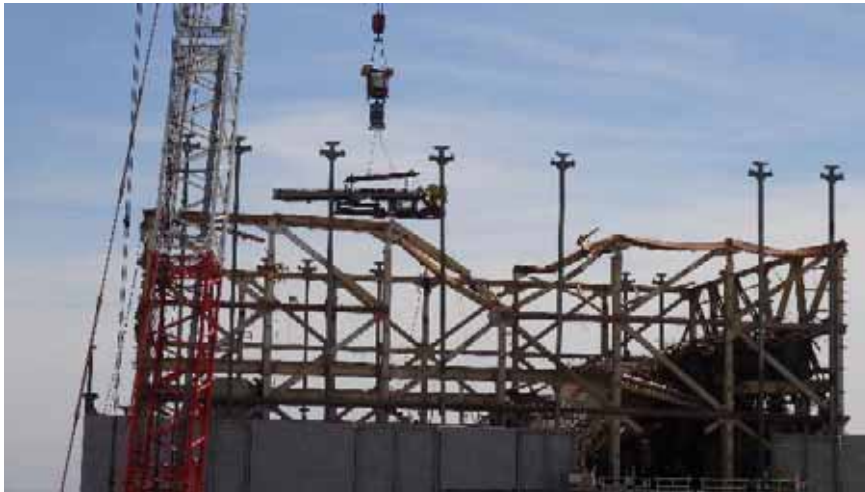
2. Hoisting cover bag insertion equipment (Photo taken on June 7)
