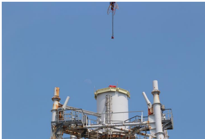
<After installing the lid>
