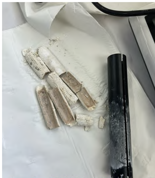
Heater protection tube and carbonate deposit inside it
