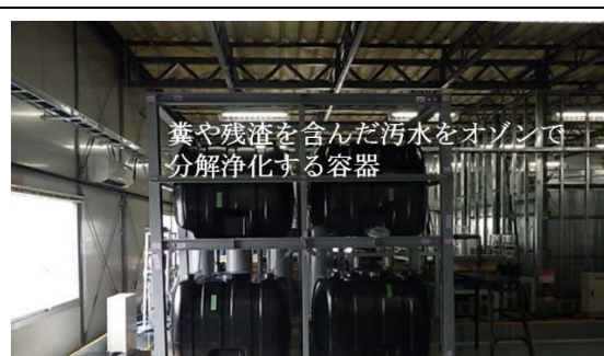
Containers for decomposing and purifying seawater containing extremot or residue with ozone
