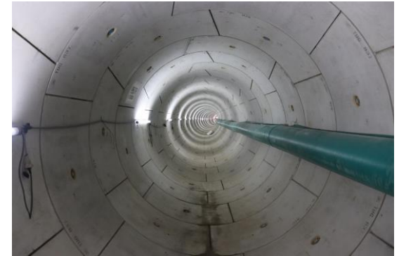
Inside of the discharge tunnel after excavation (May 2023)
