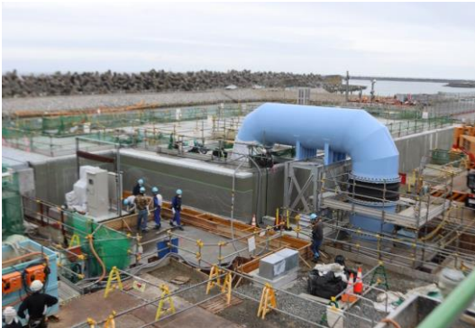
Overall view of the discharge vertical shaft (upper-stream storage) (June 2023)
