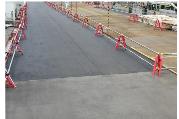
② Asphalt paving completed (September 2023)
