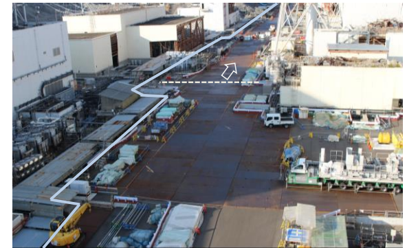
① After surfacing (Steel plates laid on top of asphalt): Wide view (February 2024)
