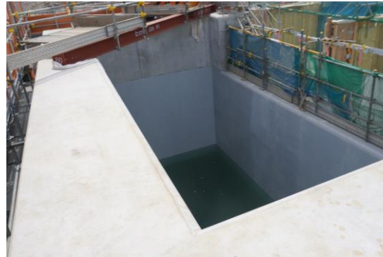
Discharge vertical shaft (down-stream storage) after being filled with water (June 2023)
