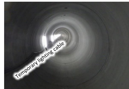
Completion status of drainage channel propulsion tunnel
