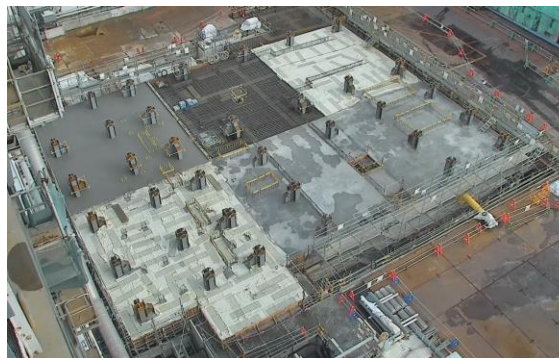
Unit 2 reactor building south side yard (gantry foundation work)
