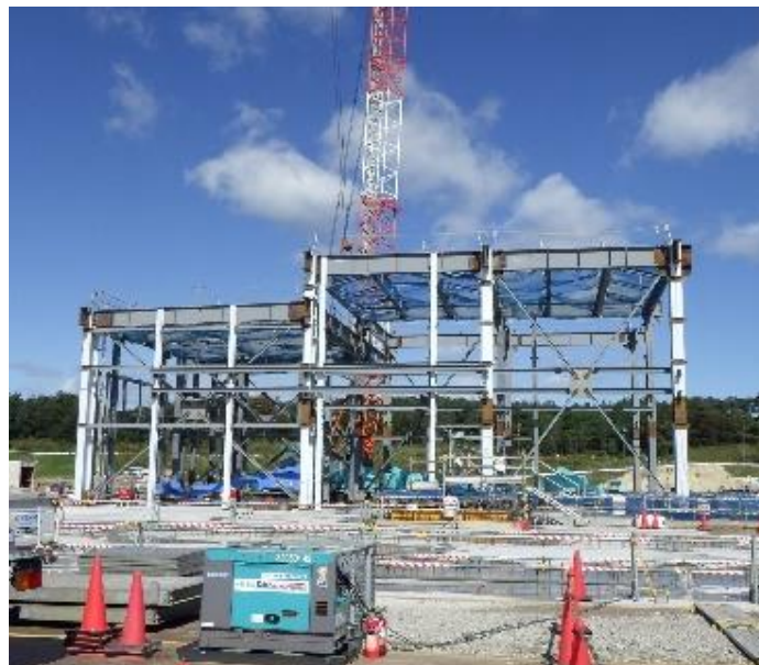
Waste volume reduction facility being constructed (photo taken in October 2021)
