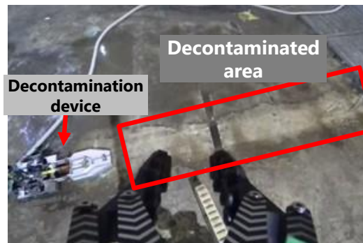
Decontamination of the top most floor of the Unit 2 R/B
