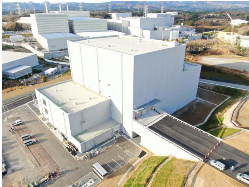
Overview of the additional miscellaneous solid waste incineration facility building
