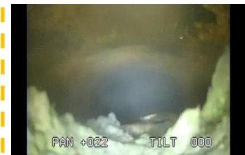
Photograph: Deposits in the X-6 penetration hole
