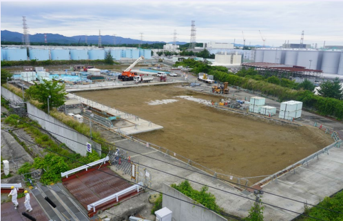
< E area after D1 tank was dismantled (photo taken on June 15, 2026) >
