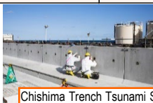
Chishima Trench Tsunami Seawall complete
