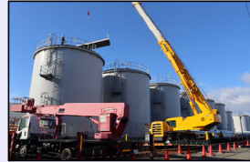
<Removing the top lid in J9 area tanks (February 14)>
