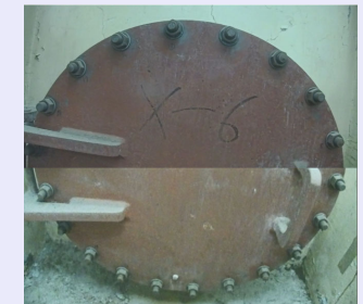
< Photo of X-6 penetration >
