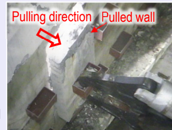
<Work to pull down the wall>
