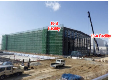
10th Waste Storage Facility
