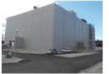
Radioactive Waste Incinerator
