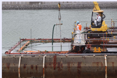
< Seafloor re-covering construction (layer of cover) >
