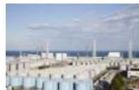
Tank area viewed from the Large Rest House (2015.10.29)
