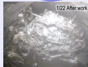
< Deposit removal by low-pressure water >
