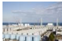
Tank area viewed from the Large Rest House (2015.10.29)
