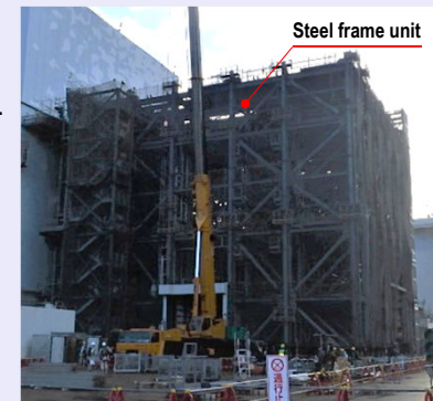
< Work on the south side of Unit 2 Reactor Building > (August 10, 2023)
