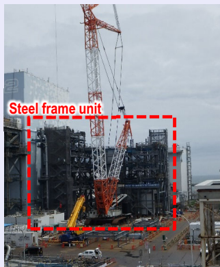
< Assembly of steel frame units (as of May 16) >
