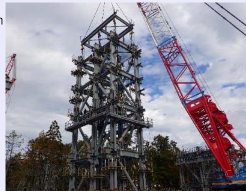
<Steel frame unit connection verification (November 5, 2022)>
