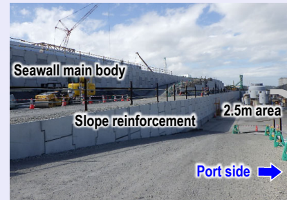
<Construction of the seawall main body>
