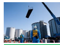
Land-side impermeable wall brine (refrigerant) circulation pipe
