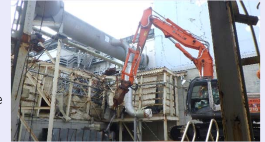
<Rubble removal work>
