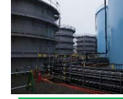
Placement of seaside impermeable walls
