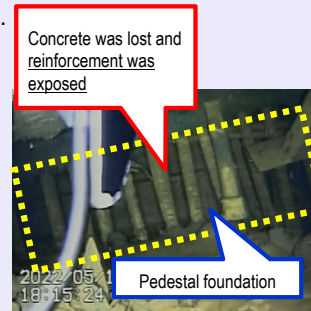
<Status near the pedestal foundation>
