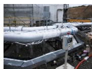
Land-side impermeable wall brine (refrigerant) circulation pipe
