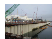
Placement of seaside impermeable walls complete
