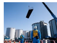
Construction of welded-joint tanks
