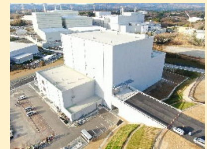
Whole view of the Additional Solid Waste Incinerator Building
