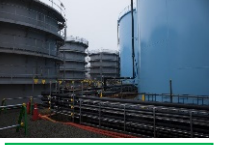
Placement of seaside impermeable walls complete
