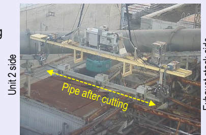
<Pipe cutting work>
