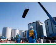
Land-side impermeable wall brine (refrigerant) circulation pipe
