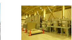
Sub-drain purification system
