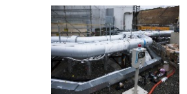
Land-side impermeable wall brine (refrigerant) circulation pipe
