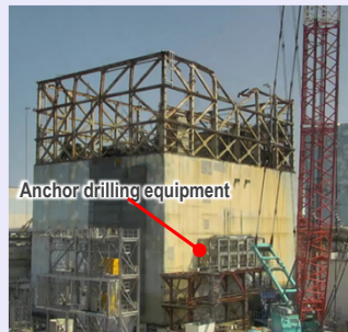
<On-site status (from northwest)> (photo: April 12, 2022)
