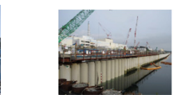
Placement of seaside impermeable walls complete
