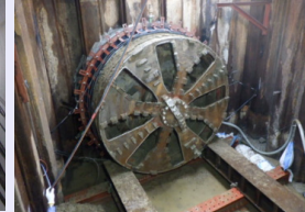
<(2) Upstream side propulsion pipe reached>
