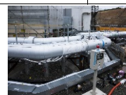
Land-side impermeable wall brine (refrigerant) circulation pipe
