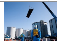
Construction of welded-joint tanks
