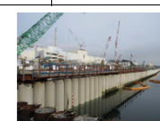
Placement of seaside impermeable walls complete
