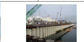
Placement of seaside impermeable walls complete
