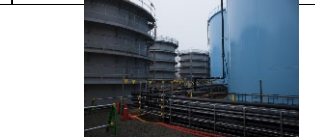
Flanged and welded-joint tanks
