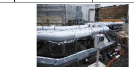
Land-side impermeable wall brine (refrigerant) circulation pipe
