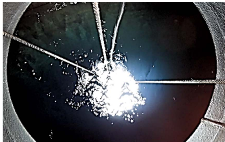
Water surface in the tank while the agitator is in operation (Picture shot at T/R)
