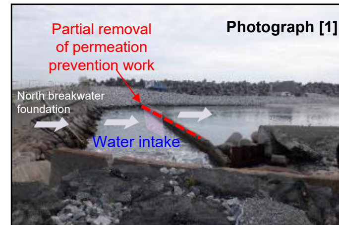
Outline of removal of permeation prevention work
