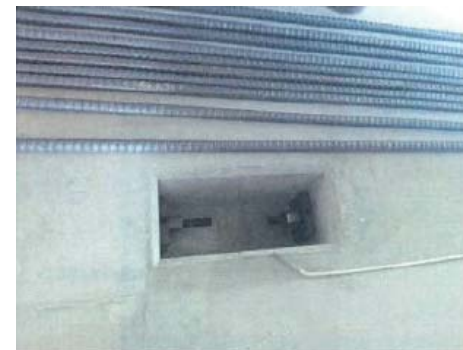
Notch filled with mortar
