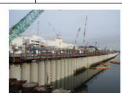
Placement of seaside impermeable walls complete
