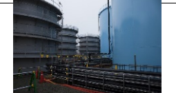
Flanged and welded-joint tanks
