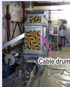
<Installation of equipment>
