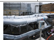
Land-side impermeable wall brine (refrigerant) circulation pipe
