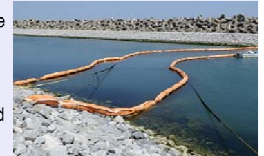
<Unit 5 and 6 open intake channel Extension of the existing silt fence>
