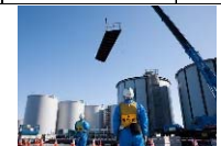
Construction of welded-joint tanks
