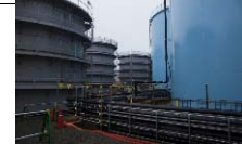
Flanged and welded-joint tanks
