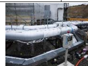
Land-side impermeable wall brine (refrigerant) circulation pipe
