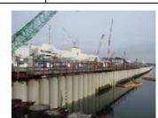
Placement of seaside impermeable walls complete
