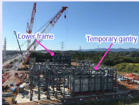
<Whole view of the yard outside the site (October 11, 2021)>
