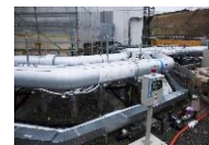
Land-side impermeable wall brine (refrigerant) circulation pipe
