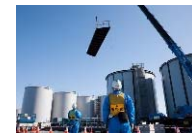
Construction of welded-joint tanks
