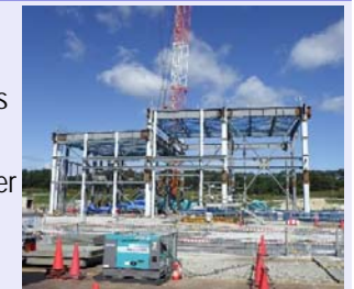
<Construction status (October 20, 2021)>
