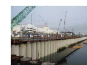
Placement of seaside impermeable walls complete
