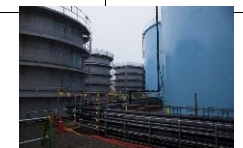
Flanged and welded-joint tanks
