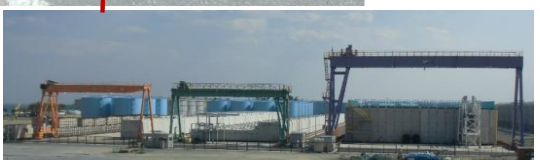
Spent adsorption vessel temporary storage facility
