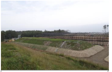
Temporary soil-covered type
