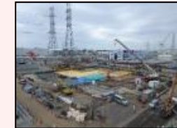
After dismantling in H1 east area
