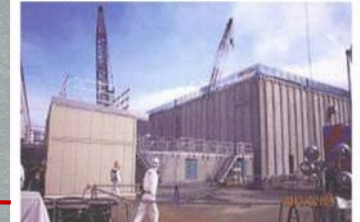
Temporary waste sludge storage
