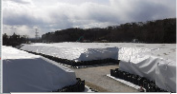
Rubble (outdoor accumulation)
