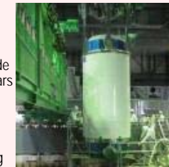
Fuel removal status
