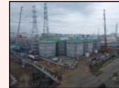
Start of dismantling in H1 east area
