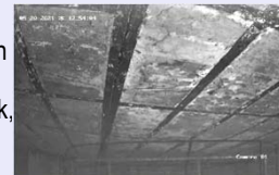
<Condition under the shield plug>
