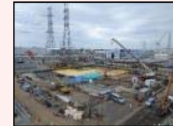
After dismantling in H1 east area
