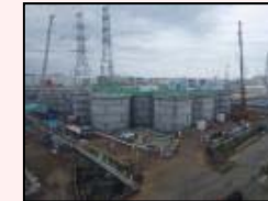
Start of dismantling in H1 east area
