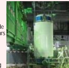
Fuel removal status
