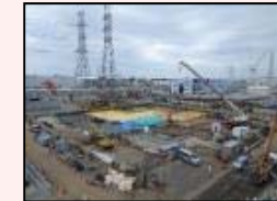
After dismantling in H1 east area
