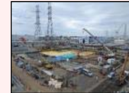
After dismantling in H1 east area
